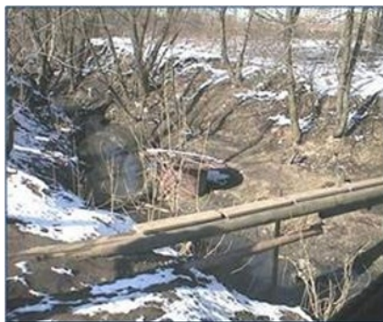
Fig. 6. Zhuzha River before rehabilitation project (2005).
